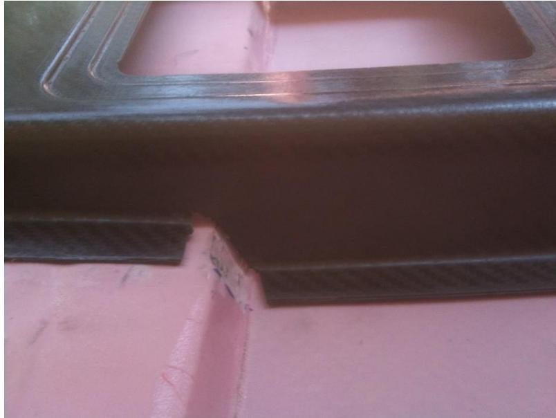
While fitting the console to the cabin top, use clamps and clecos to hold everything in place. Do NOT drill through the cabin top, just drill deep enough for the cleco to have some bite.
